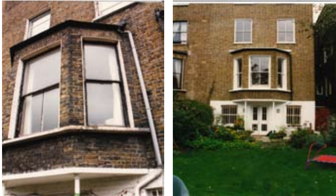
Rear elevation before and after rebuilding and new windows
