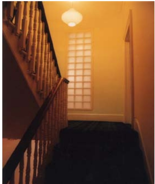
View up staircase to borrowed light from bathroom
