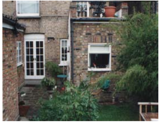
View from garden before work
